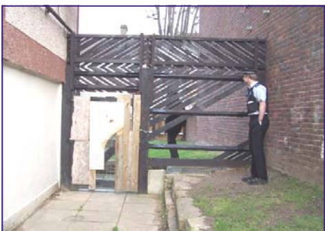
This gate and fence will be replaced with a metal version
