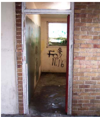
Caretakers cupboard to be boarded up
