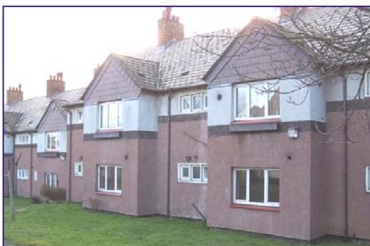
Back of properties which have been broken into
