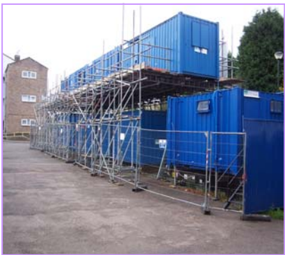
Breyer's site office and storage area
