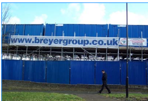
Breyer's site office and storage area
