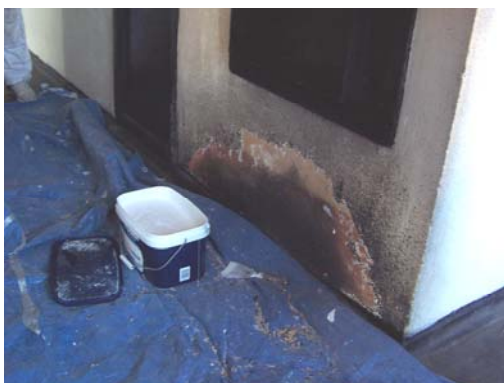
Repair work is being carried out
