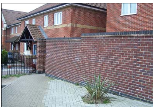
The wall by Rosewood Court
