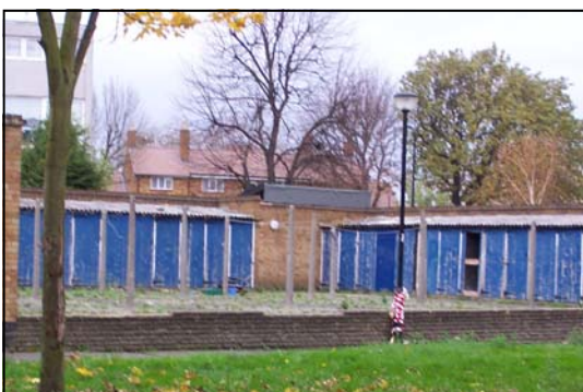
Sheds which have been damaged
