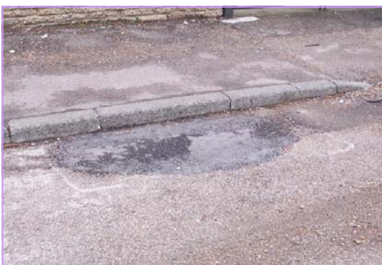
Potholes have been filled
