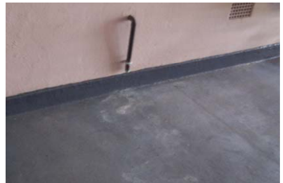
Lime scale residue which is difficult to remove in the drying area
